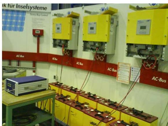
Fig. 29: Two three phase Sunny Island 4500 battery inverter clusters at the DeMoTec with connected Haag measurement devices (see section 4.1.4)
