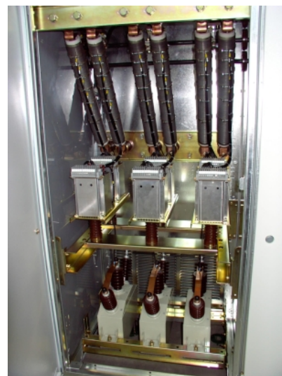
Fig. 28: Line impedance with switchable R, X and C
