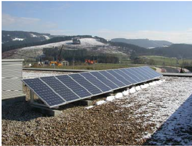
Figure 3-3: Mono-crystalline structure based photovoltaic installation
