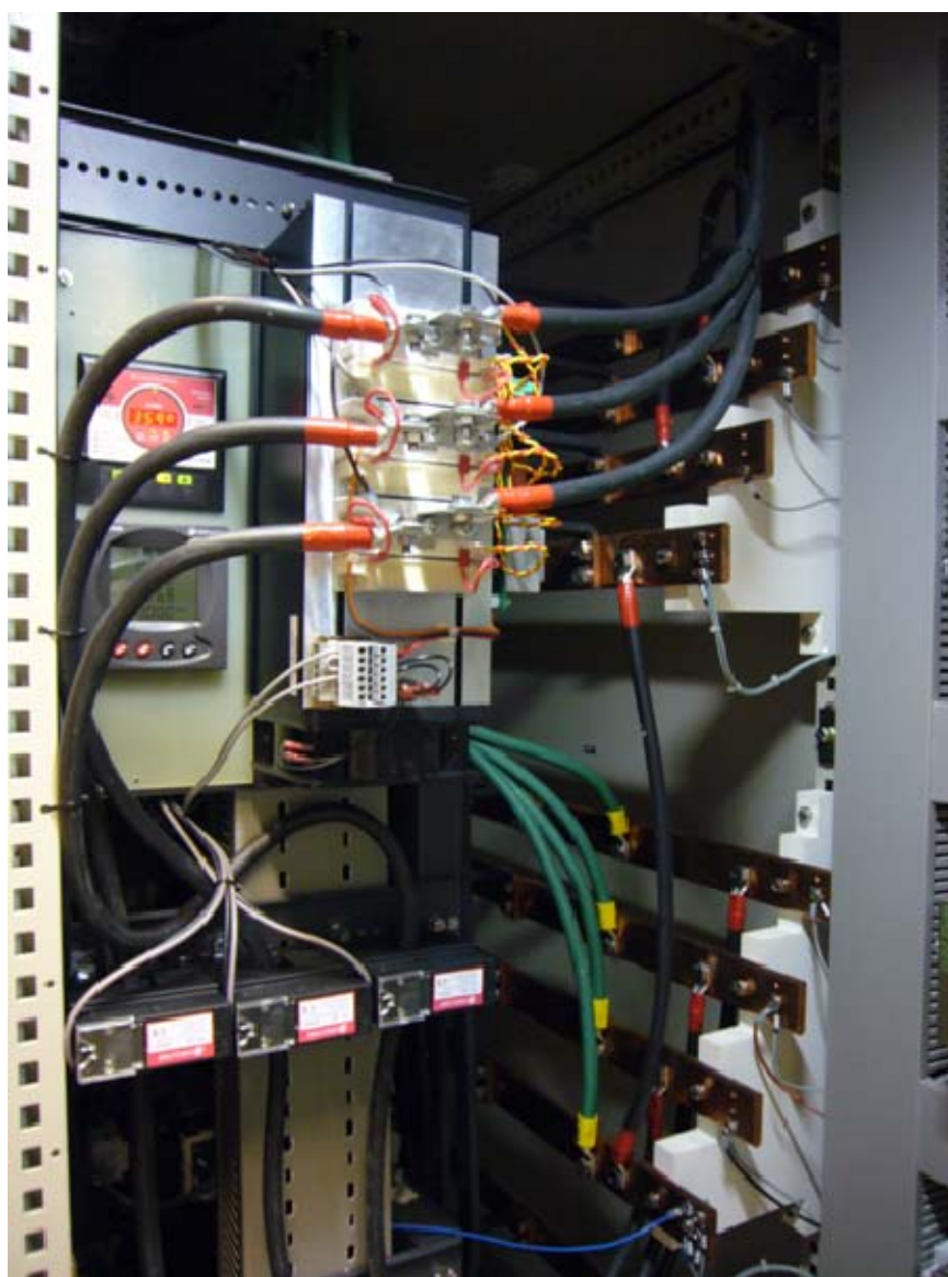
Figure 2-5: Detail of the static switch
