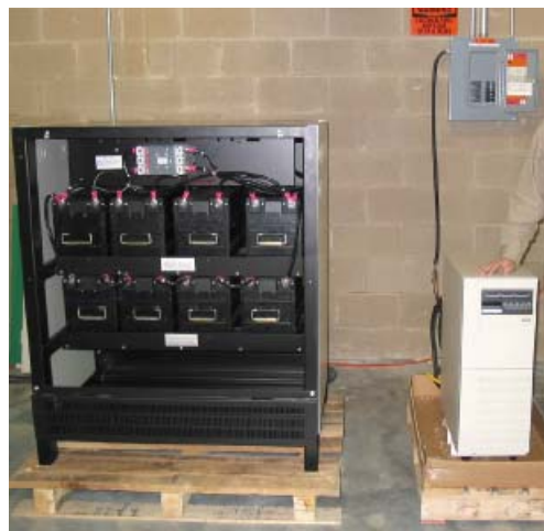
Figure 3-9: Ultra capacitors bank
