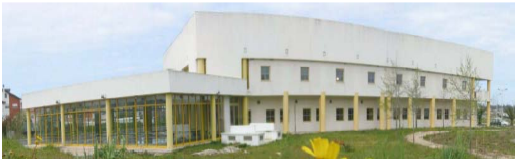
Figure 1 – External view of the Ílhavo MSP building
