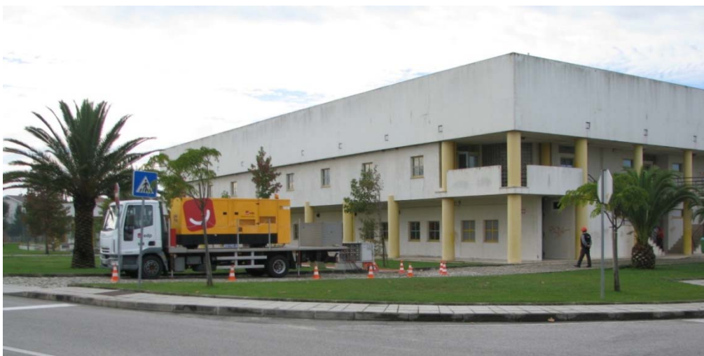
Figure 97 – Overview of the Ílhavo MSP during the field tests
