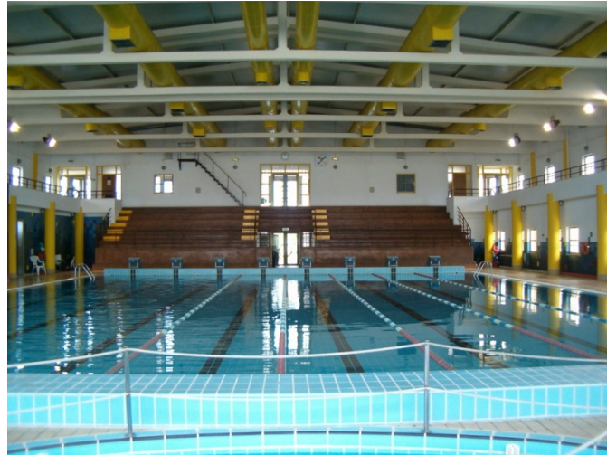
Figure 2 – Inside view of the Ílhavo MSP – Main tank
