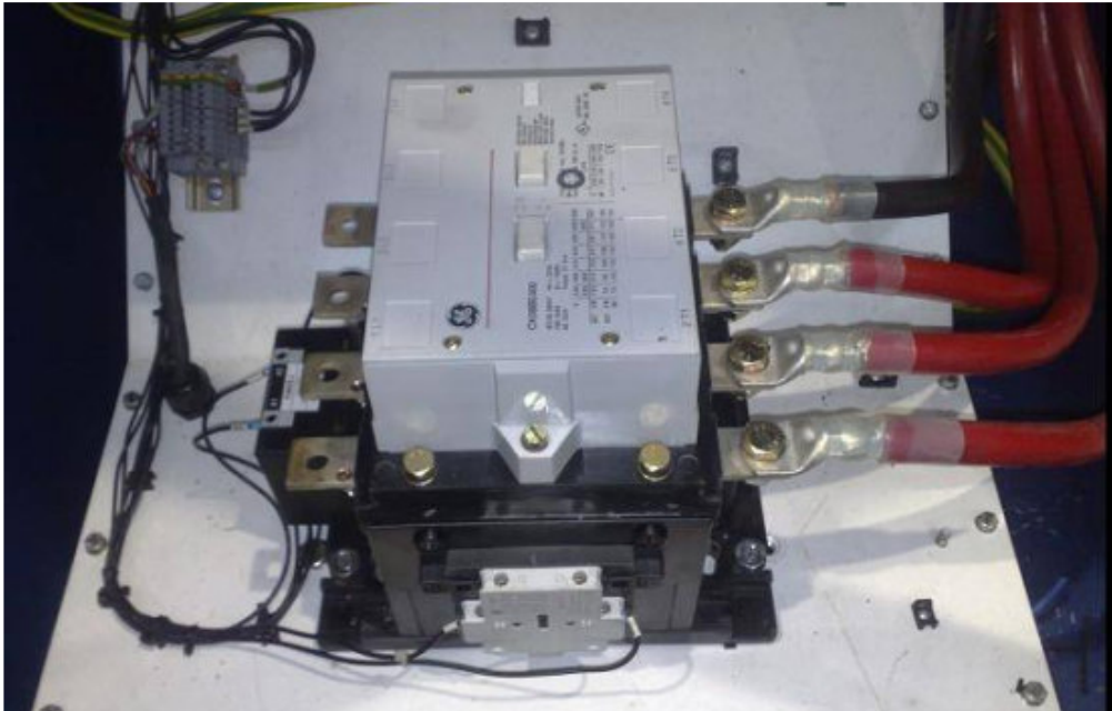
Figure 2.9 – Contactor C (bypass breaker).
