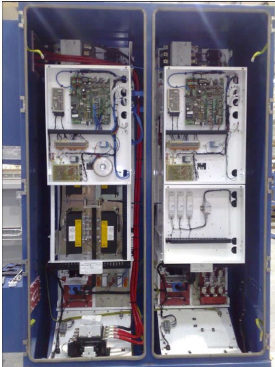
Figure 2.4 – Inside View of the I-Power ENT200 Converter
