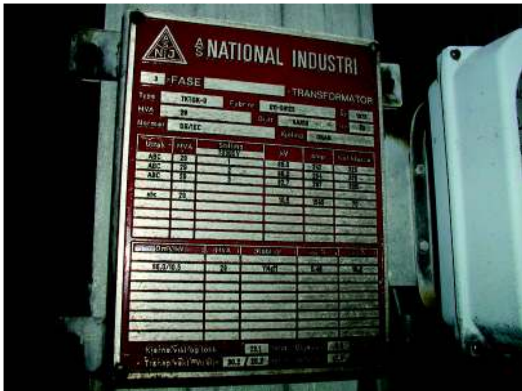
Figure B.3: Nameplate from step-up transformer in unit 5
