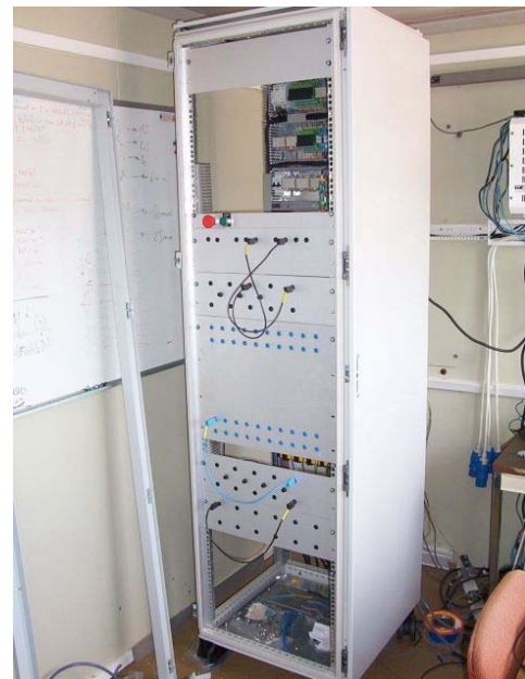
Figure 78: Front face of the main cabinet (under construction)
