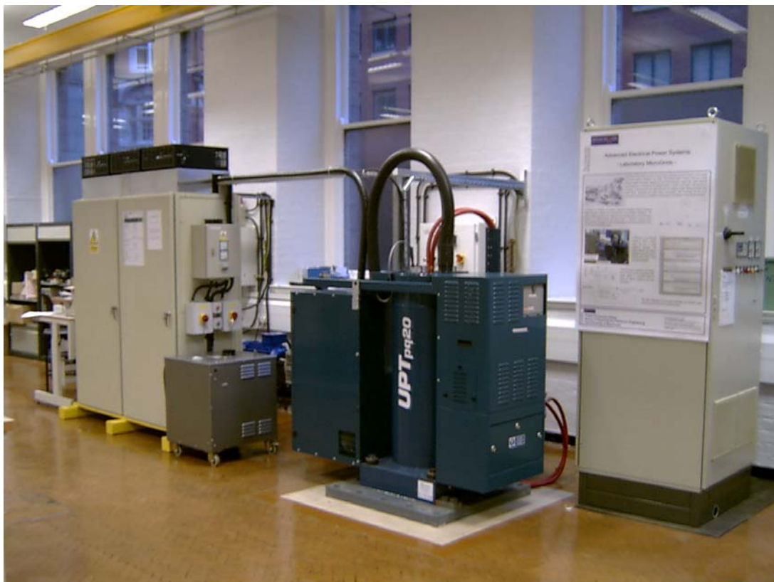
Fig. 53: May 2005 – Completed hardware
