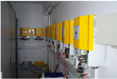
Fig. 5b: Sunny Island inverters
