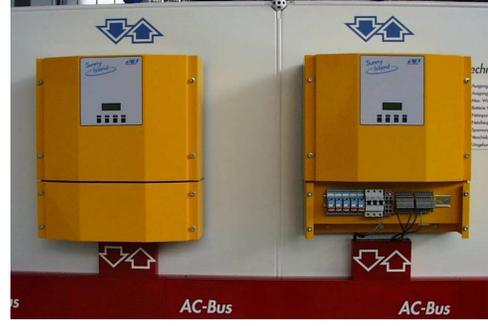
Fig. 4. Two battery inverters *SunnyIsland*<sup>TM</sup> by SMA Regelsysteme GmbH, Kassel, Germany operating in parallel (rated power 4.2 kW, clock 16 kHz, coupling inductor 0.8 mH)
