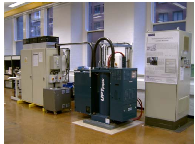
Fig. 7: View of flywheel installation
